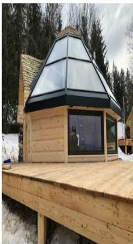
Fig 16. Example of previously built Cabins
