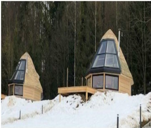
Fig 15. Example of previously built Cabins
