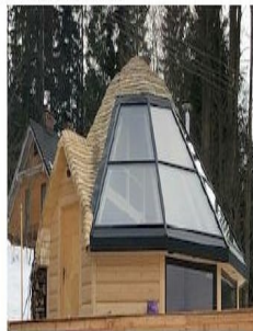
Fig 17. Example of previously built Cabins
